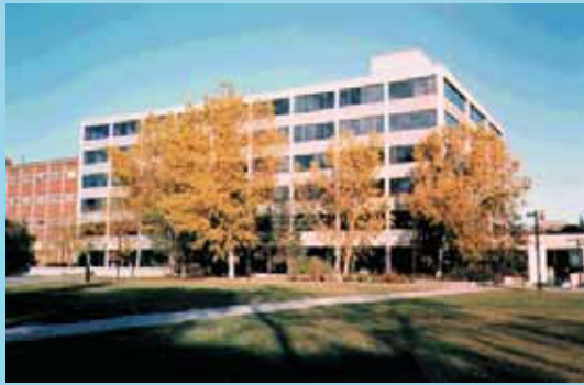
Central Academic Building, PIMS-UA Site Office.
