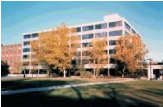
Central Academic Building, PIMS-UA Site Office
